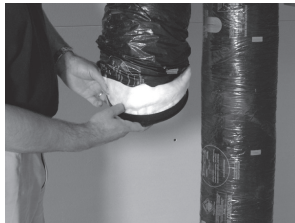
Insert insulation inside the double collar.
