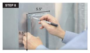
8. Use the included metal frame to trace the outline onto the duct. Allow for a 1/8" space around the marking as to allow the frame to sit properly in the duct. The duct opening window should have the following dimensions: 8.5" x 5.5".
