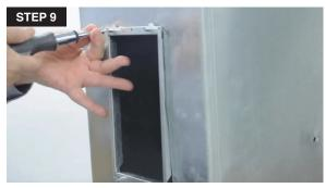
9. Place the frame into the opening made in the duct and use the 6 metal screws provided in the installation kit to secure it in place. Use preferably 3 top and 3 bottom holes of the frame to insert the screws.
