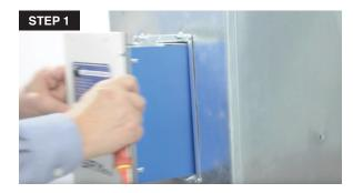
1. Take the SR Max out from the ductwork by removing the 4 screws located on the cover (4 corners) that hold it to the frame.
