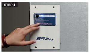
4. From now on, the SR Max will only activate the lamp when the thermistor detects airflow in your duct system.
