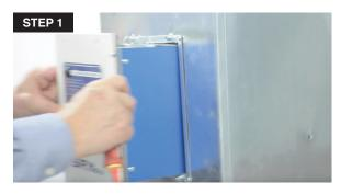
1. Take the SR Max out from the ductwork by removing the 4 screws located on the cover (4 corners) that hold it to the frame
