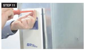
11. Secure the SR Max to the frame with the 4 remaining screws located in the 4 corners of the SR Max cover.
