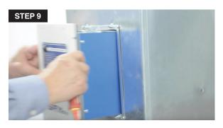
Once the new UV lamp is installed, replace the SR Max into duct.
